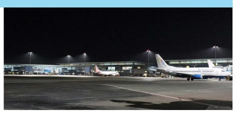
A customized dimming system is incorporated into the system that adds further savings. The dimming system allows each pole to be grouped into 'zones' and/or controlled individually. During slower periods of the night, the lights are scheduled to dim down to 50% intensity to save on electricity costs.
