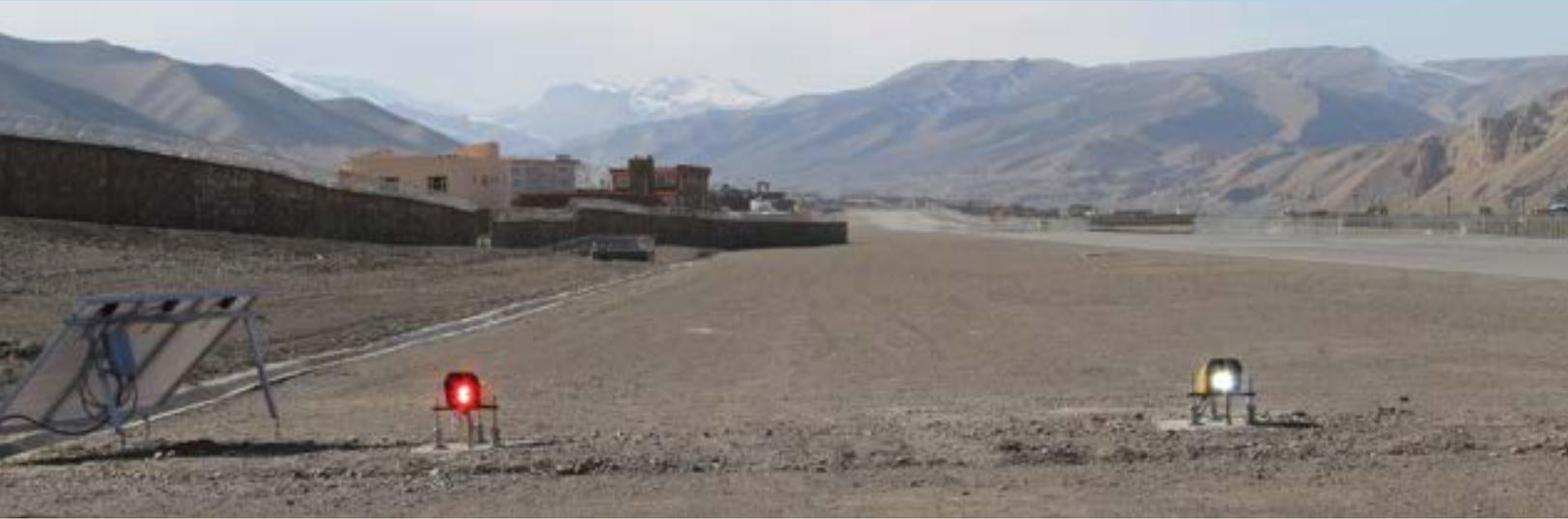
This project presented a challenging feature with a fence line located right along the safety zone, thereby requiring a highly efficient solar system to operate the Solar Series LED PAPI while eliminating any other possible alternatives. With the civil works completed, Aviation Renewables completed the installation of the Solar Series LED PAPI's and MAPPS hybrid power system within two days.
