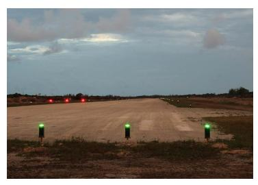
the lights to be relocated, the lights were unbolted, moved and installed without the need for cabling or trenching. Each light being self-contained ensures redundancy and reliability of operations according to ICAO standards.
