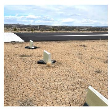
The bases, however, were still in good condition and could remain in place. The airport sought help from Aviation Renewables to design, manufacture and deliver new retroreflective sheaths in order to continue using their existing marker bases.
