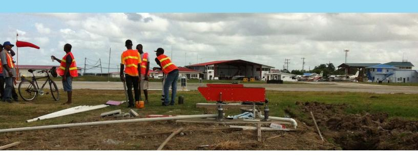
The Solar Series wind cones incorporate an FAA LED L810 with photocell control and a Solar Series RMS engine for self contained operation, easy installation and no maintenance over the next 5 years. Working with Aviation Renewables, the installation for the solar LED airfield lights and Solar Series wind cones was achieved within days.
