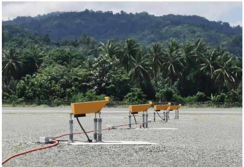
Aviation Renewables has supplied multiple solar powered LED PAPI systems to this region to support temporary, semi-permanent and portable LED runway lighting operations. Using these easily transported systems enables the airport operator to provide continuous, safe and ICAO compliant LED PAPI operations for jet traffic during periods of airfield construction, runway resurfacing projects or any unexpected events of power failure.
