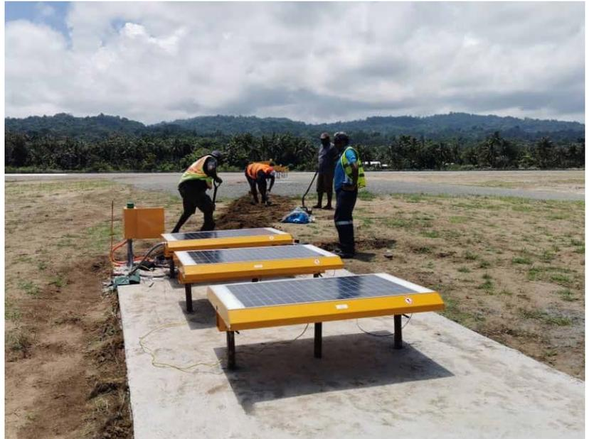
The L854 Pilot Activated Lighting Controller is integrated into the PAPI Power Control Unit and maintains a passive listening watch on the aerodrome frequency. When the L854 detects 3, 5 or 7 clicks on the VHF frequency, the unit instructs the PAPI to illuminate in low, medium or high intensity, respectively.
