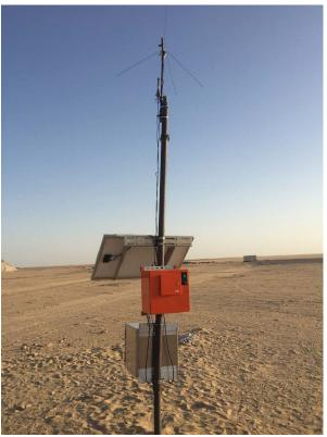
With proper use, the solar LED runway lights are anticipated to operate for 5-7 years with zero maintenance, at which point the battery will need to be replaced. With timely battery replacements, the anticipated service life for the system is 15-20 years.
