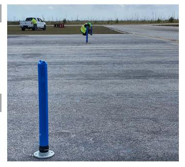
As part of the rebuilding process, the airport elected to use Solar Runway Edge lighting. These self-contained lights were installed at a lower cost than conventional lighting and are IP68 waterproof to prevent damage from any future damage from seawater at the low-lying airport. Due to the limited budget that the airport was allocated for re-construction, they were eager to find ways to save money while still offering a fully ICAO-compliant lighting system for night operations.
