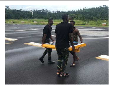
The solar LED TLOF lighting is activated by a pilot activated radio controller, which allows the pilot to use the VHF radio in the cockpit to control the intensity of the lighting. The lighting is standalone and autonomous, requiring no connection to grid power or electrical wiring. Aviation Renewables was on site to lead the installation and commission the system. The entire system was installed and operational within 5 days.
